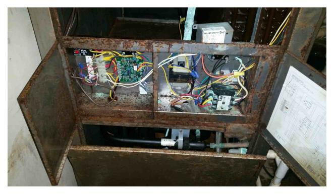
This dehumidification system was destroyed by corrosion resulting from poor pool chemistry
