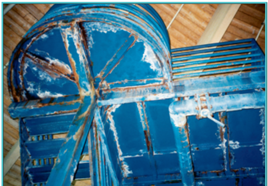
Corrosion under this waterslide stairwell indicates the facility's mechanical systems are not properly controlling such pool environmental factors as air and water temperature and relative humidity.
